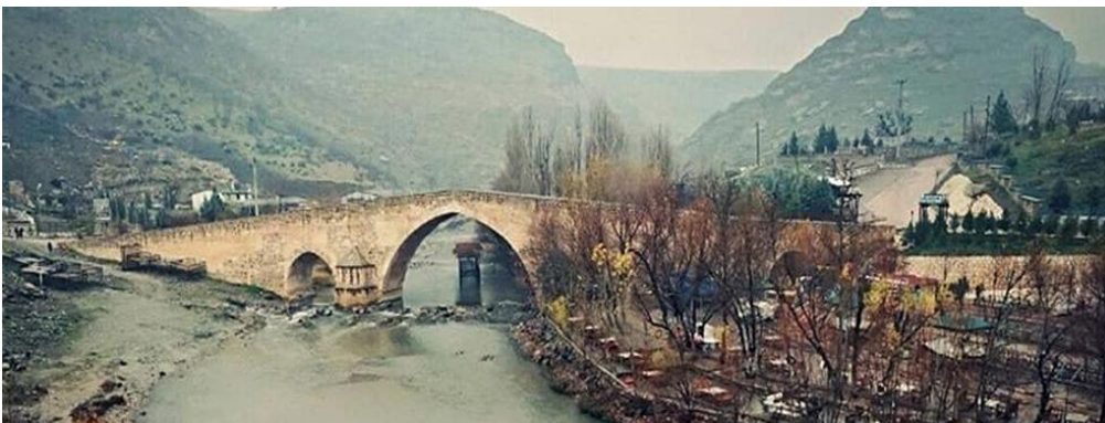
Figure 4. Haburman Bridge (MoCT, 2024)
