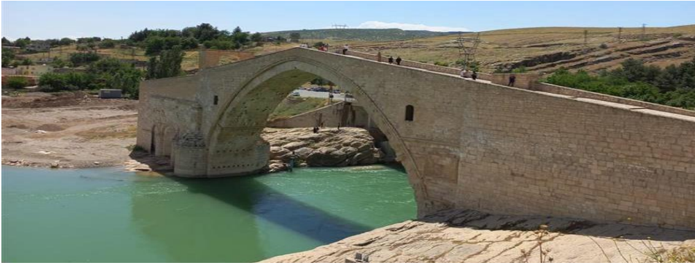
Figure 3. Malabadi Bridge (MoCT, 2024)
